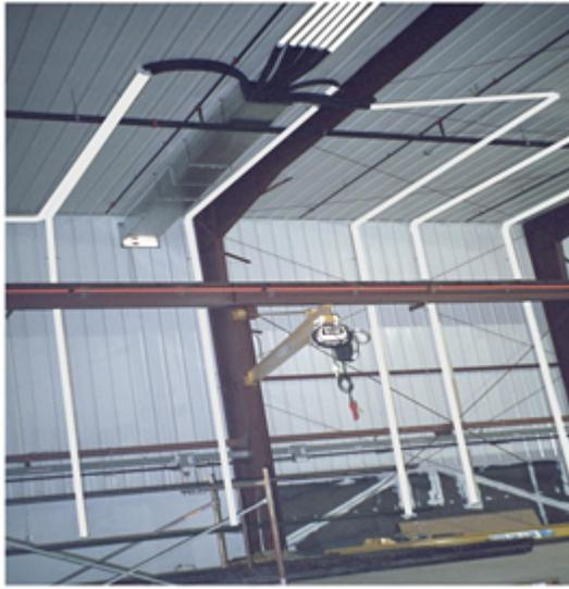
**10. Install second section of duct work.** Couple 10' sticks of corrugated tubing the same way tubing is attached to head of system.
